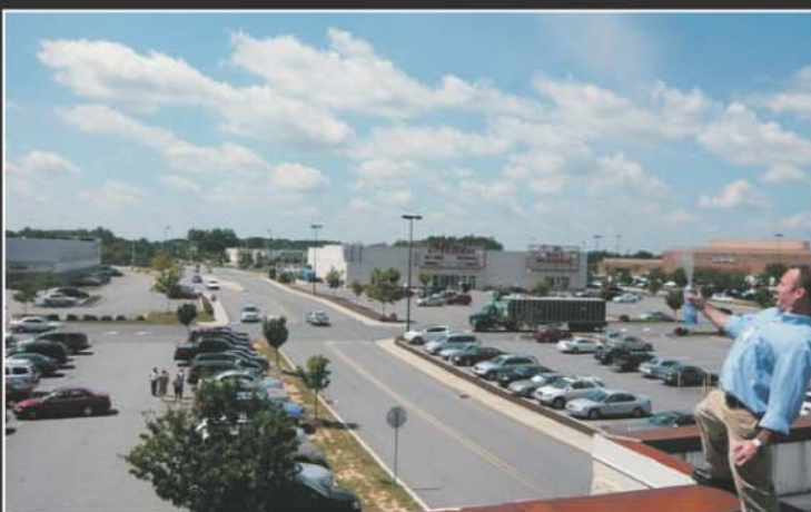
Roof top air direction
